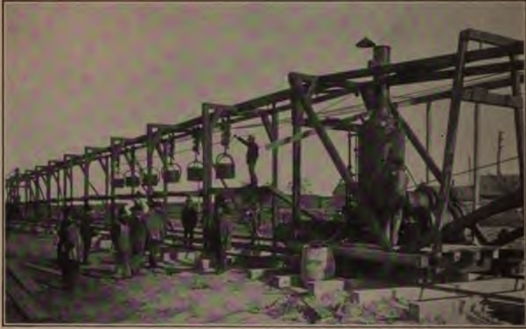
"Carson-Trainor" Trench Excavator on Sewer Trench Construction. Figure 121.
